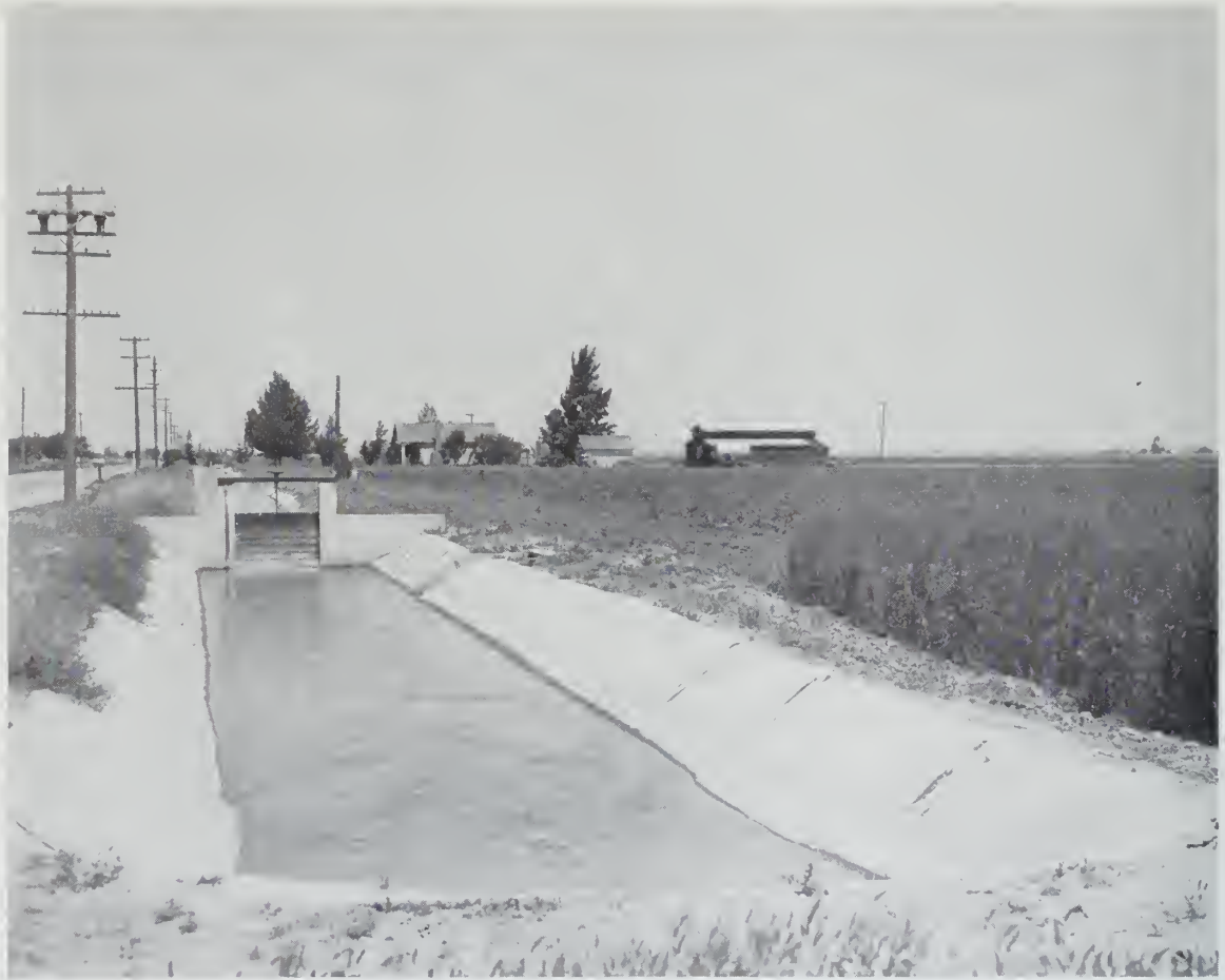
Canal Conveying Irrigation Water in Western Mokelumne Unit
